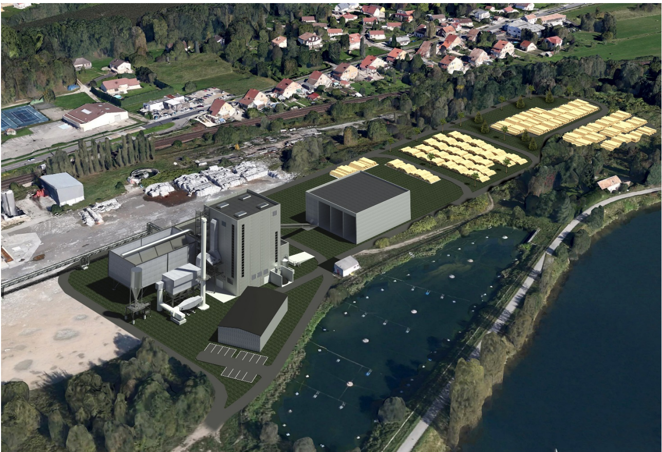
The CHP plant Cogénération Biomasse de Novillars is situated on the site of the papermill Gemdoubs.
